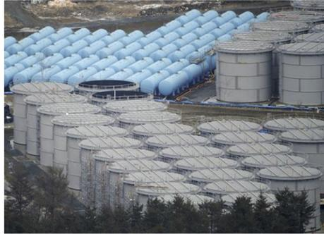
**Fig. 1.** Tanks in the Fukushima Daiichi Nuclear Plant. The tanks are used to store contaminated water.
